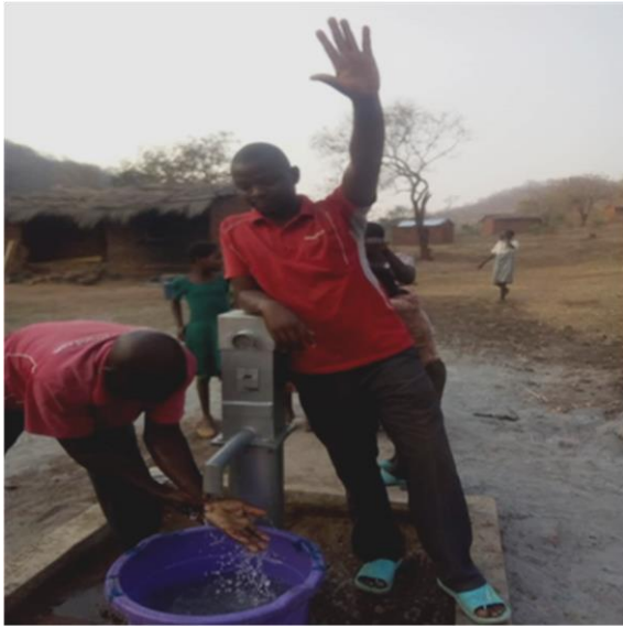
SHADRECK LEANING ON THE NEW HAND PUMP
